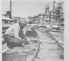
WELDER'S torch cuts once-shining rails into convenient lengths for striping. TORCH of welder ta corta e riel den pizanan grandi pa worde benta afór.
